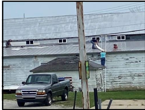
West side of building gets new windows, steel roofing and siding. Next will be the east side.
