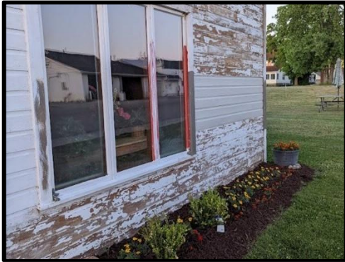
Front face of our building being blasted, scraped and readied for paint. Flowers planted.
