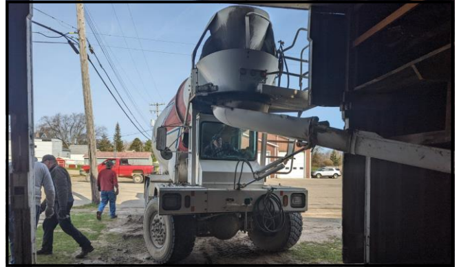
Cement being poured in the bay areas.
